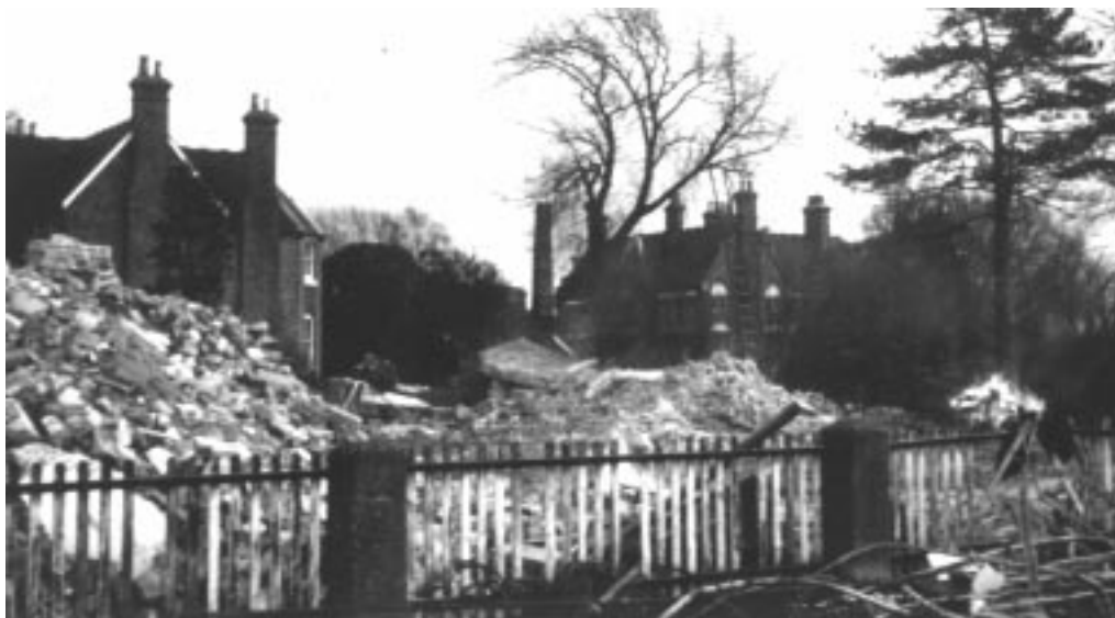
Demolition in progress 1965 Photograph courtesy of Kitty Wheatley
