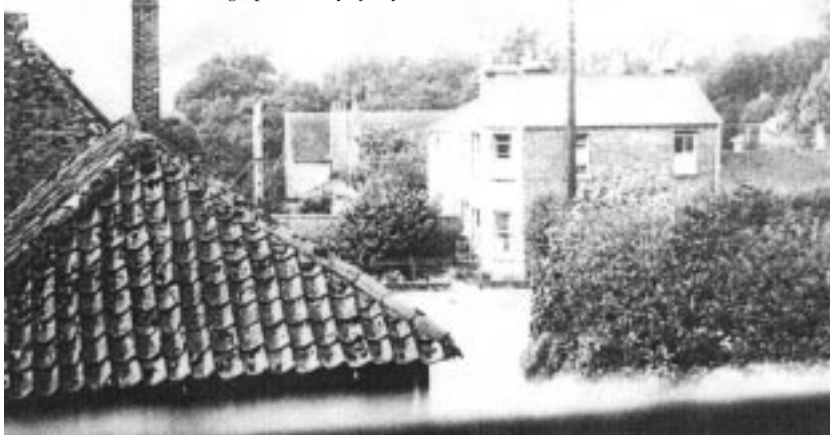
The roofs of Old School Cottage and its barn on the left and, in the distance, the roof of the forge to the right of Forge House Photograph courtesy of Ivy Burnett
