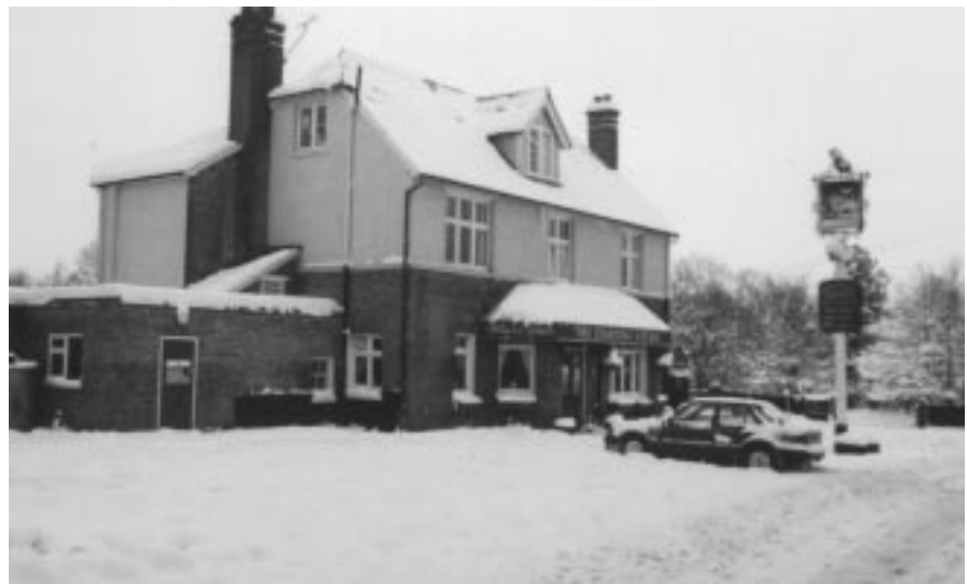
The Fighting Cocks building has changed little over the years Photograph courtesy of Trevor Manning
