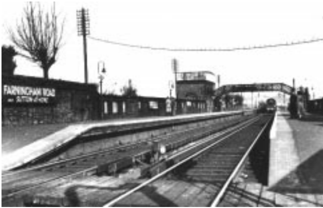
The station in 1953 Photograph courtesy of R C Riley
